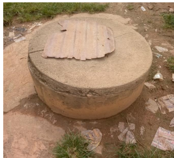
Figure 7: Self-help hand-dug well in Ayetoro Source: Authors' fieldwork, 2023
